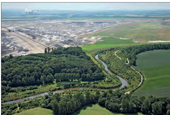
Fig. 5: In the background: Inden mine and Weisweiler power station; in the foreground: recultivated land with the relocated Inde river
